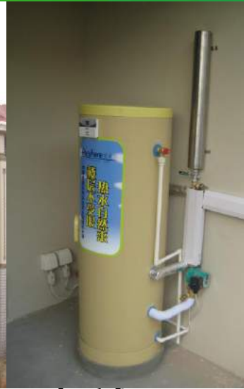
Balcony split solar hot water project for Qingdao Yixinyuan community
