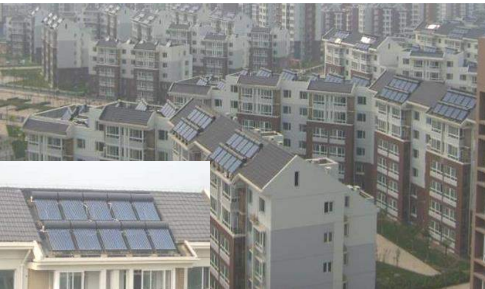
Solar hot water project for Huaming Town government, Tianjin
