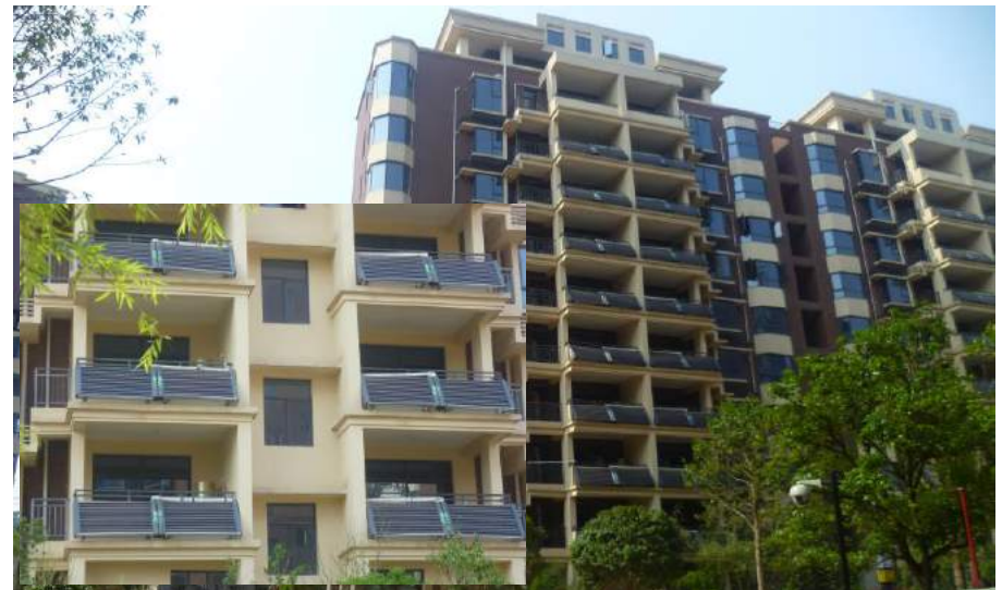
Balcony split solar hot water project for Changsha Hanlinyuan community
