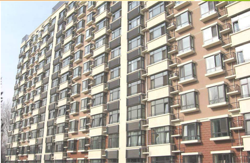
Balcony split solar hot water project for Beijing Fifth Design Institute
