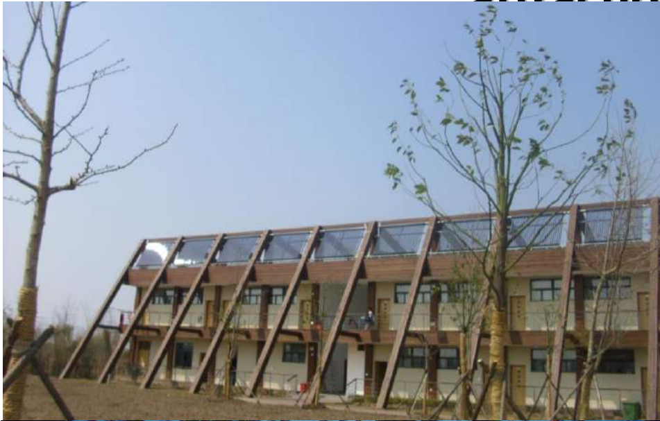
Solar hot water project for Shanghai Chongming island wetland park
