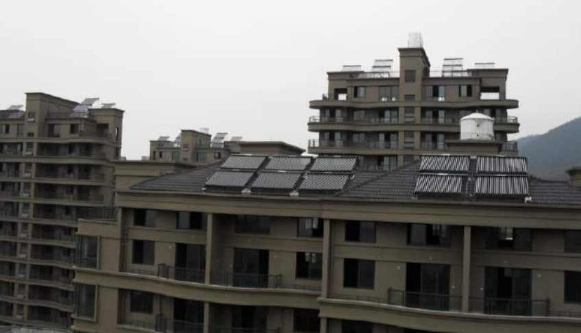
Solar hot water project for Fuyang yalin apartment in Zhejiang province
