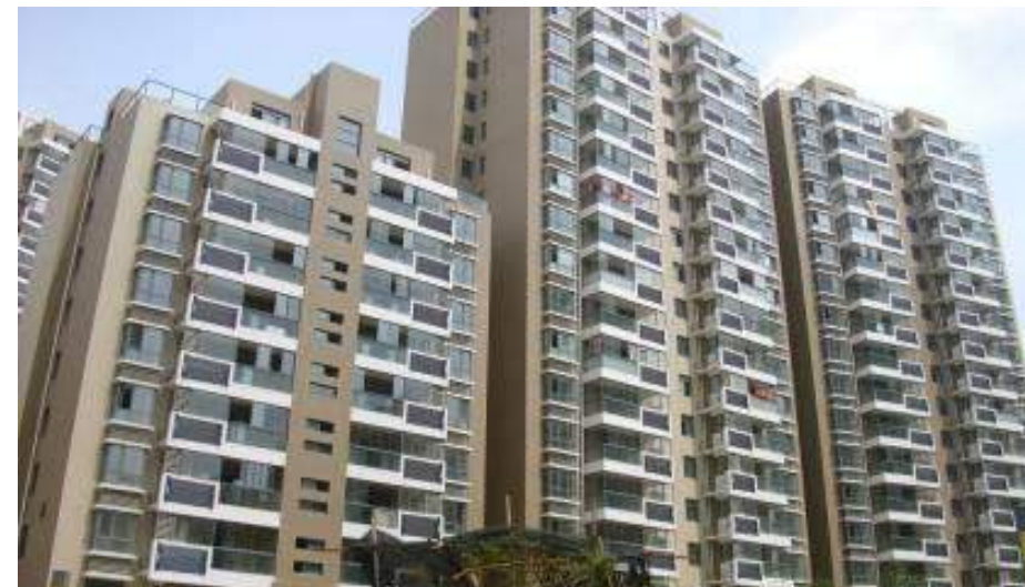
Balcony split solar hot water project for Hefei Minghang family community
